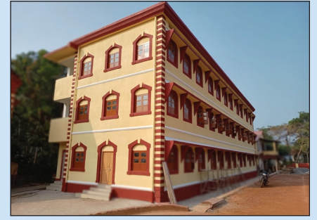
Holy Cross School, repaired and updated.
